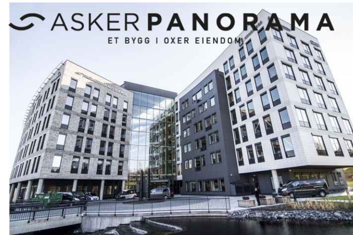
Asker Panorama 2 MW, heating and cooling run by 10 wells replacing ~250 wells*
